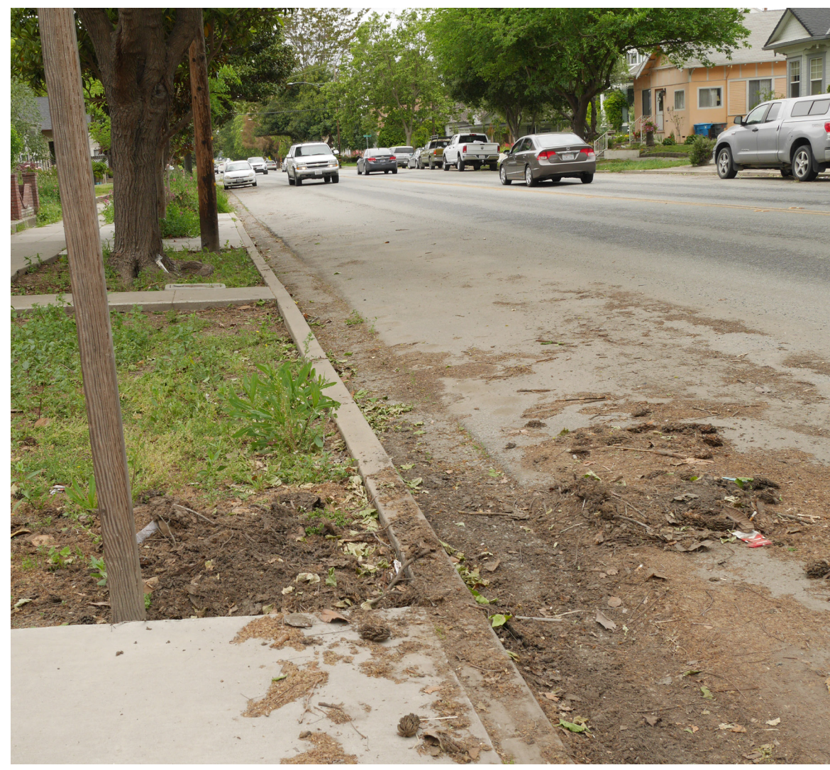
A considerable amount of sediment and debris collects along the gutter line of the street.
