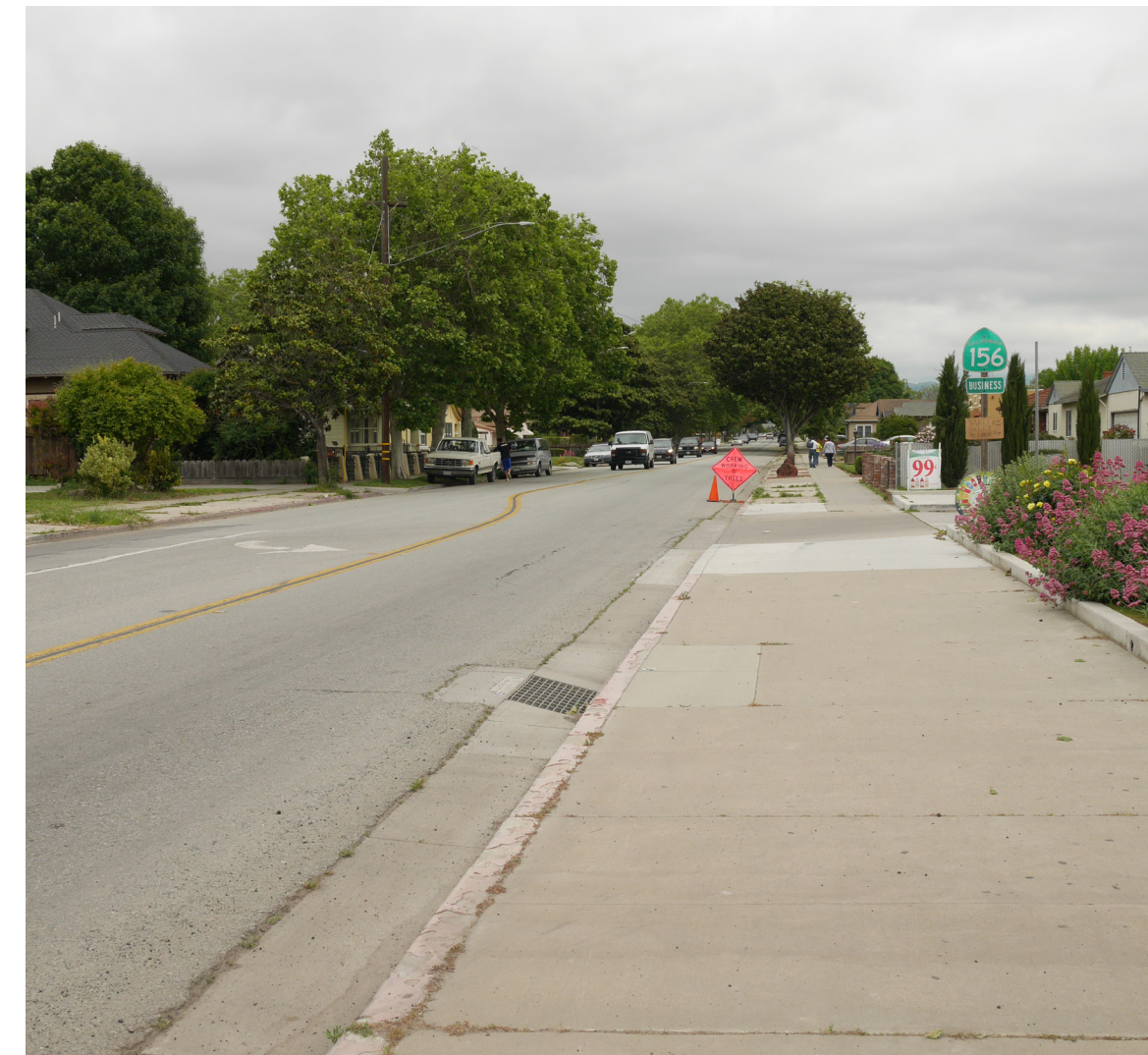
Many stretches along the 4th Street are devoid of street trees and landscaping.
