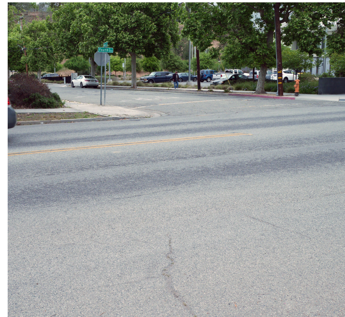
Wide pedestrian crossing distances at intersections creates difficult conditions for people to safely cross the street.
