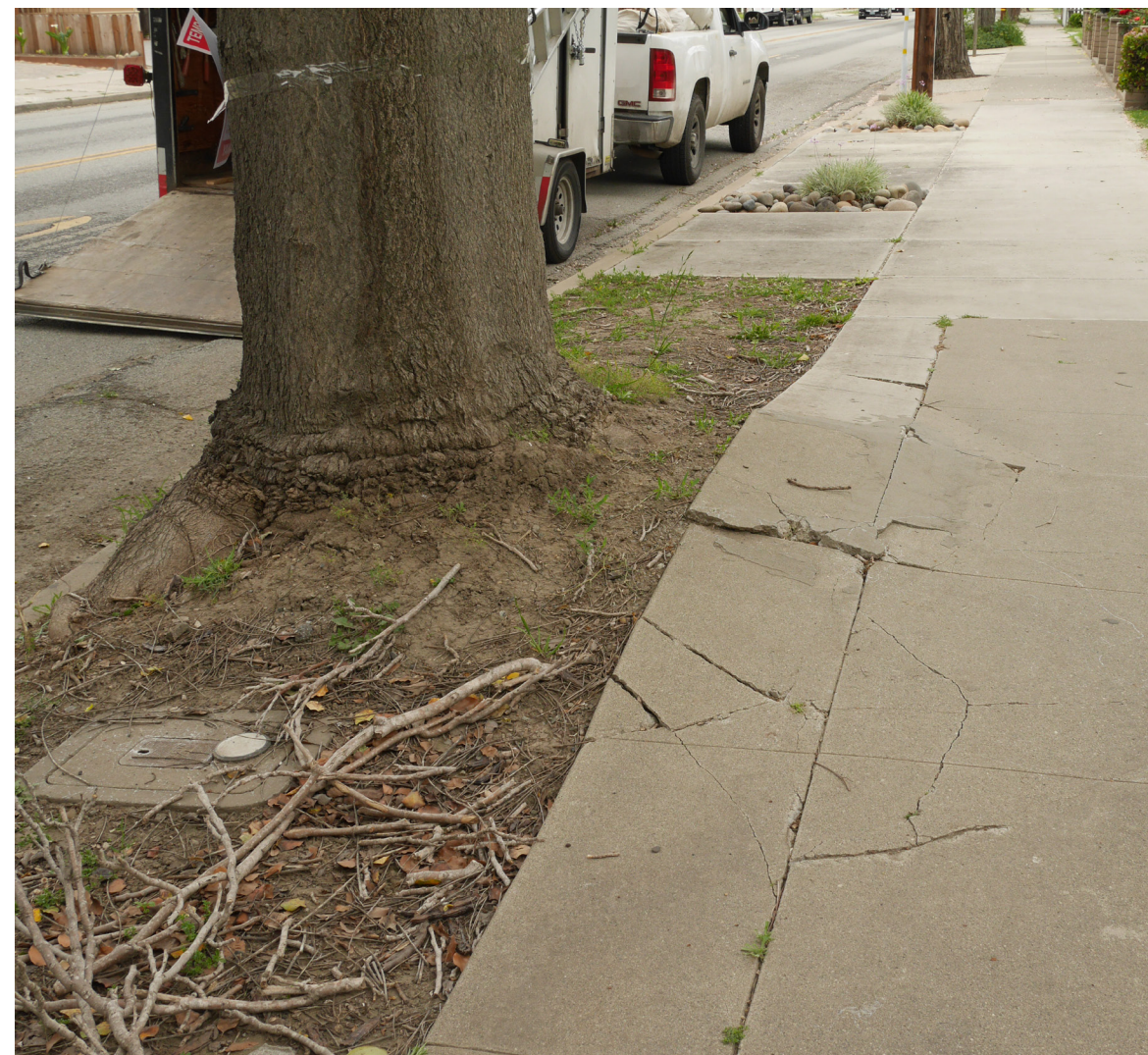
Some mature trees have outgrown their existing landscape strips and have compromised the sidewalk.
