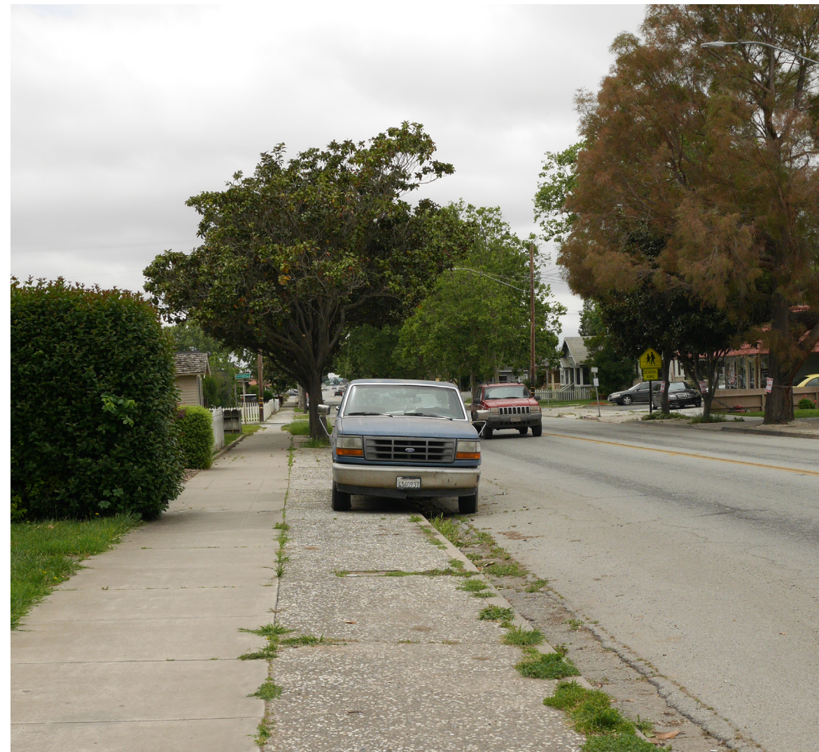
Residents often drive their vehicles over existing curbs to provide more room to park their vehicles.
